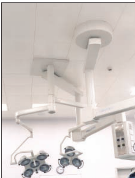
Larger ceiling tiles are important in areas where high levels of hygiene are required.
